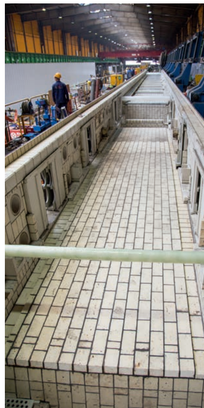
Brick lined pickling tank
