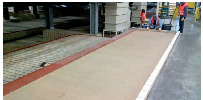
Installing a screed coating
