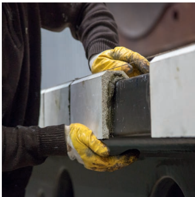
Working with synthetic resin mortar
