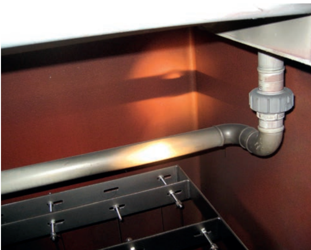
COROFLAKE coating in a wet ESP
