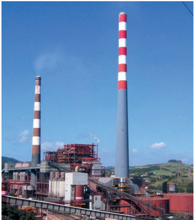
Coated power station chimney
