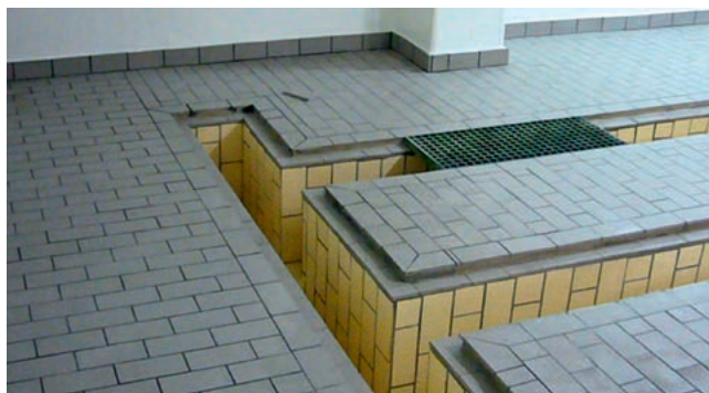
Combined covering implemented with gutters
