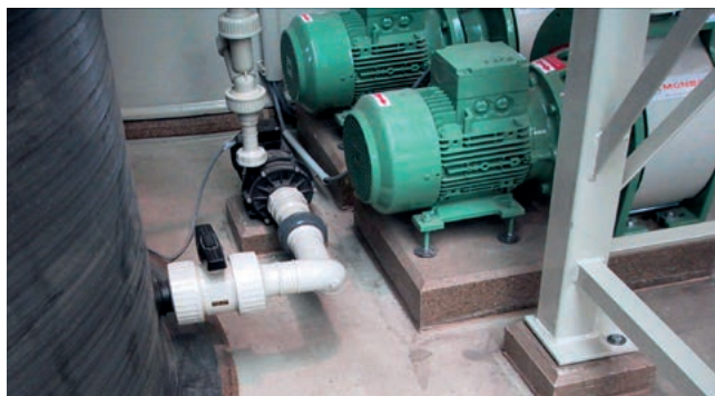
Polly-concrete bricks as pumping equipment foundation
